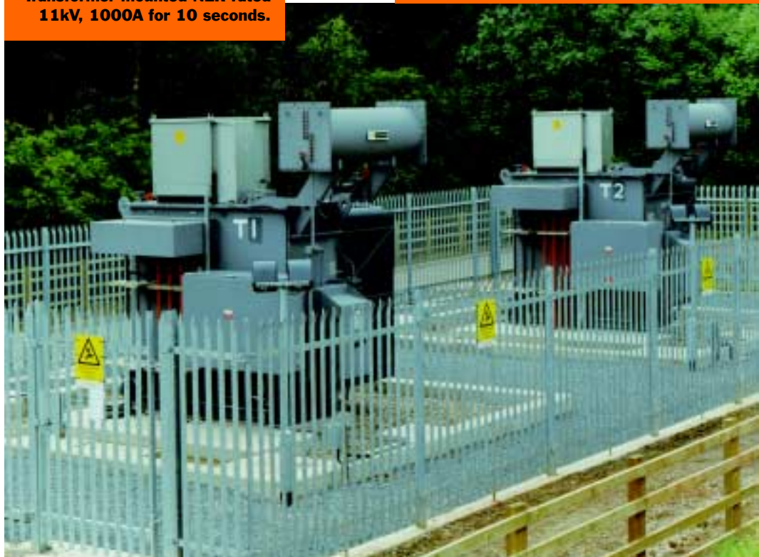
NER rated 11kV, 625A for 10 seconds installed in a substation near Heathrow.
